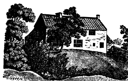
A simple but attractive dwelling with a capacious cellar.
